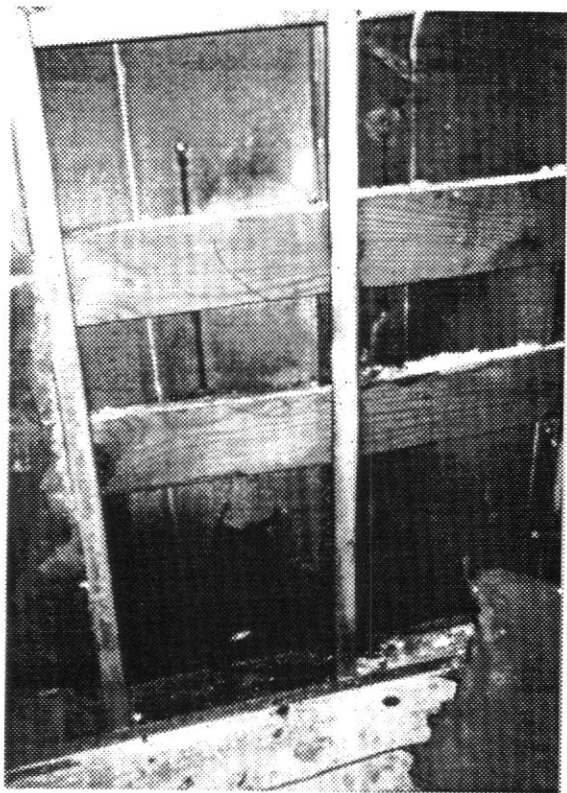
FIGURE 7 MOISTURE CONDENSATION (interstitial space)
