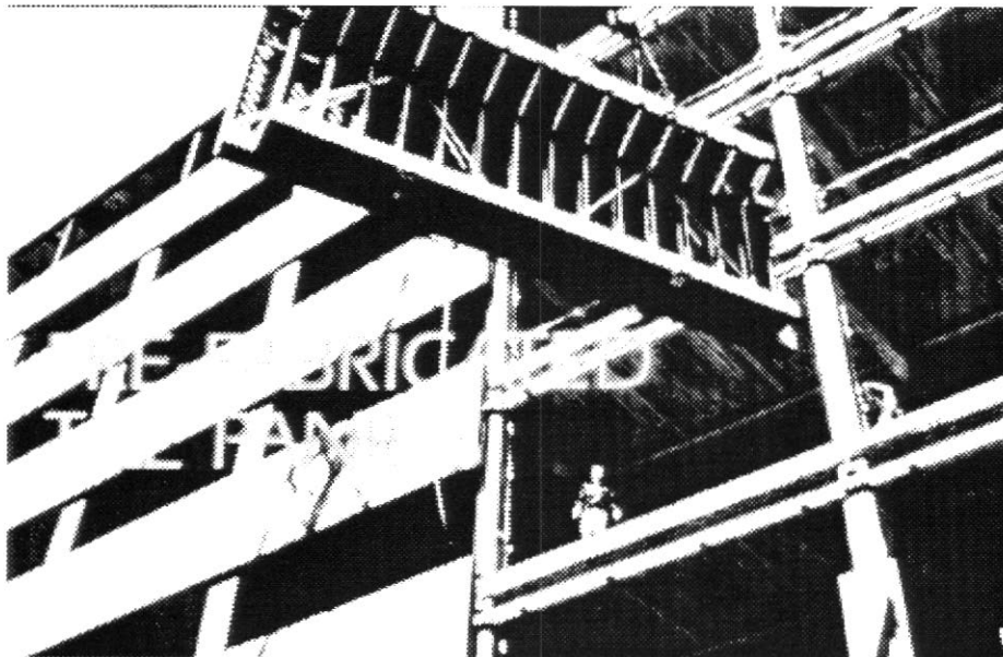
FIGURE 4a DIRECT ADHESIVE METHOD (Pre-fabricated panels)
