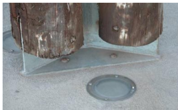
Figure 4. Column base (coexistence of different materials & technologies), PE (author's collection).
