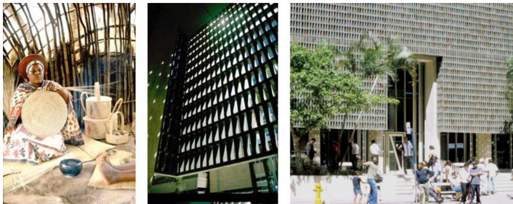
Figure 7. Ceramic façade providing environmental control - inspired by African and Islamic traditions, (author's collection).
