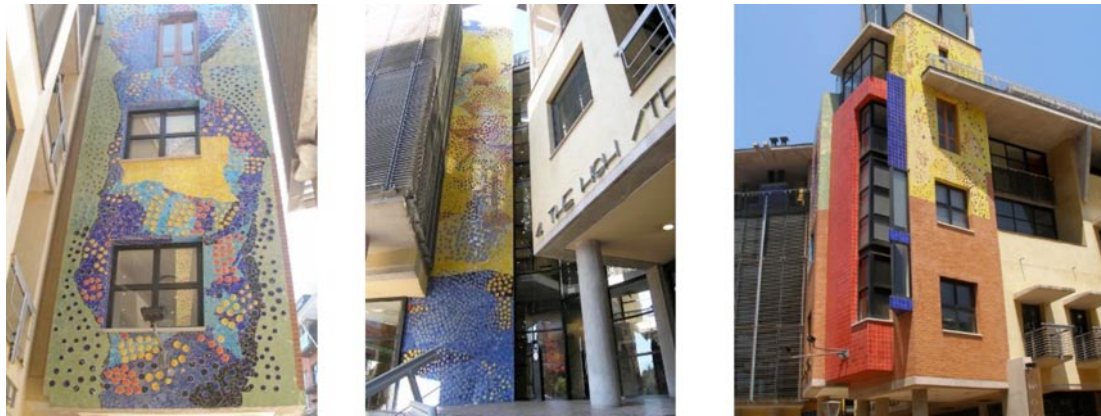
Figure 30. Local industrial and handmade ceramics installed as cladding – façade details, Jhb ( http://www.durandmosaic.co.za/Public%20Spaces.htm ).
