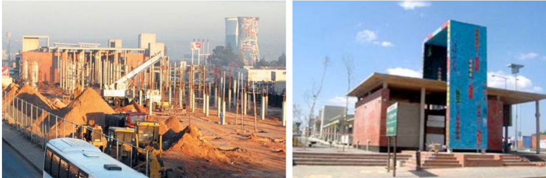
Figure 24. Baragwaneth Taxi Rank - overview ( http://joburgnews.co.za/2004/sep/bara1.jpg & http://www.durandmosaic.co.za/West%20Street%20(19).JPG ).
