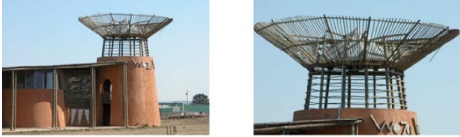
Figure 2. Concrete blocks ( representing 'developed' technology) used to build traditional Zulu oval forms) and gum poles ( the 'underdeveloped'), applied to columns, the tower and signage (author's collection).
