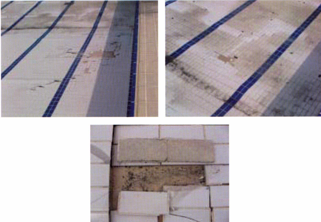
Top pictures show buckling and debonding failure of tiles in a swimming pool. The failure proliferated upon draining of the pool water for repair. Down picture shows a close up view of the mode of failure. Most of the tiles failed by cohesion fracture along the surface of the screed, indicating a poor screed quality
