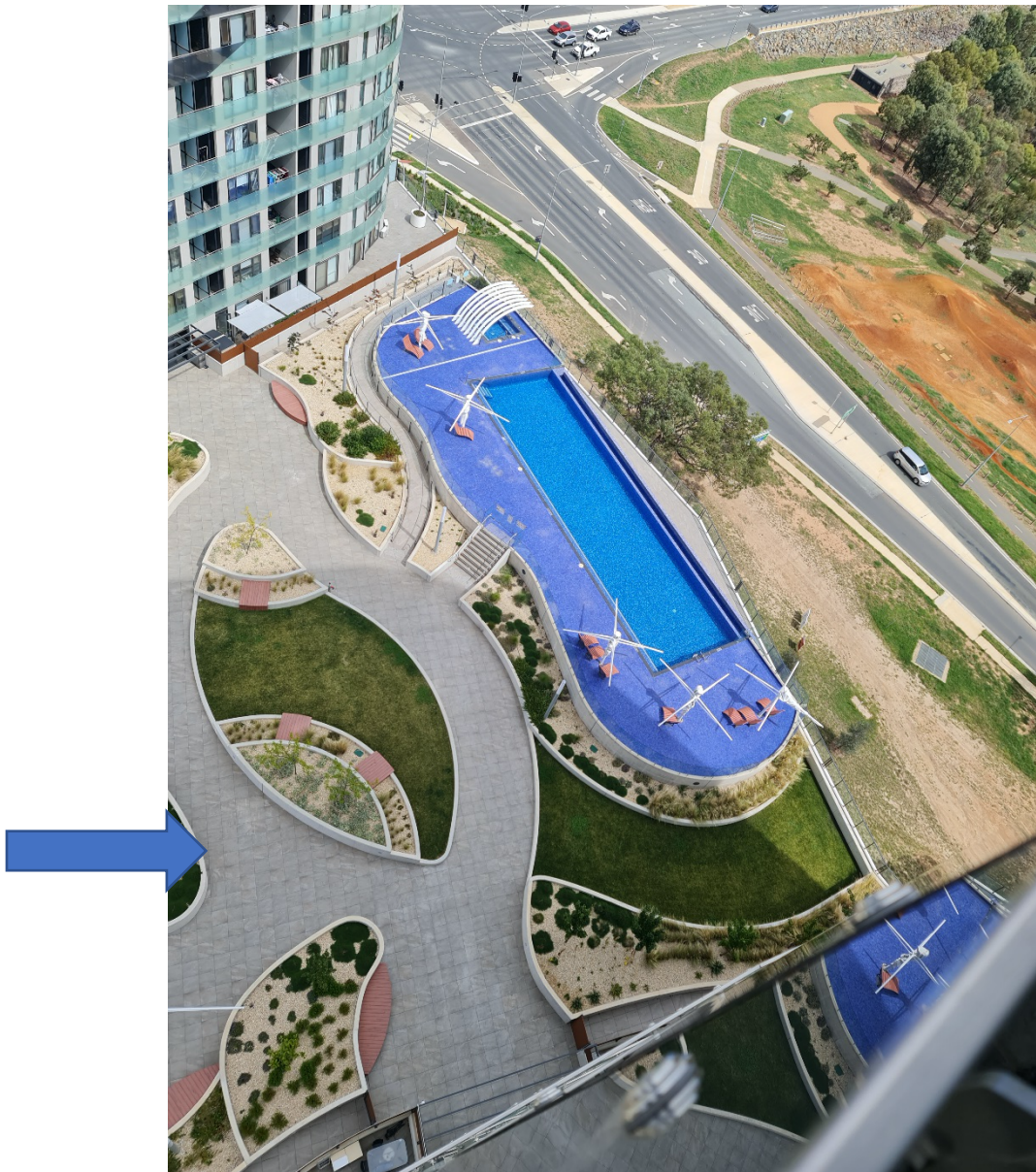
Photograph 1. Common Podium Tile installations are used in large public areas such as this 420 unit apartment block 'Sky Park' on level 5
