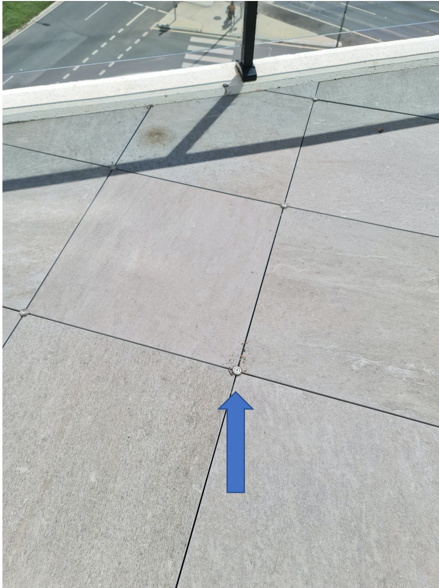
Photograph 2. depicts mechanical fixing sytem to prevent dislogement of tiles that were previously flipping over in high winds.
