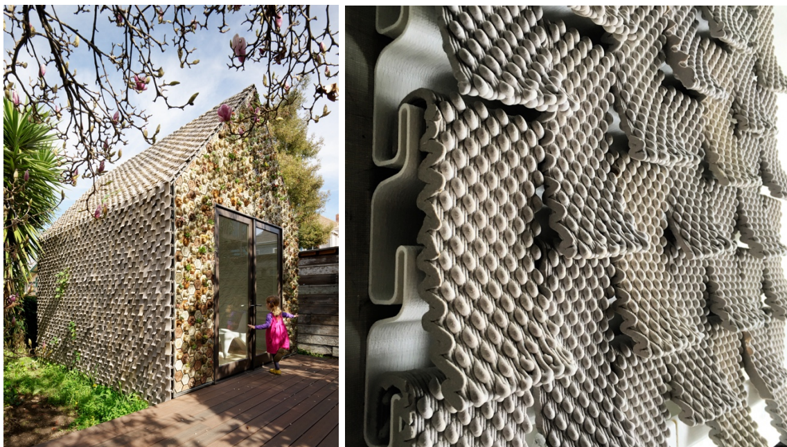
Figure 11 – 3D printed ceramic shingles clad the walls and roof of an experimental cabin.
