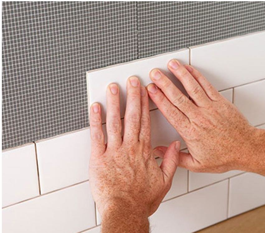
Figure 8 – The self-adhesive mat for tile installation replaces water-based adhesive and allows faster finishing.
