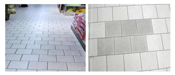
*Figure 1.* Heavy shading of the surface, leading to strong colour-transitions on the floor (left) and locally highly visible mosaic effects (right)
