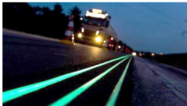
Figure 7. Highway N329 in Oss, Netherlands. Powder paint markings containing luminous particles that use sunlight to charge up during the day.
