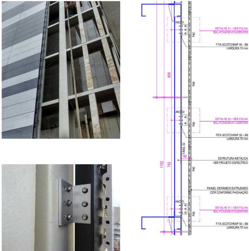
**Figure 2.** Ceramic frame in design and construction detail
