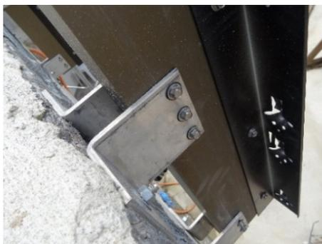
**Figure 9.** Pinned support with round holes
