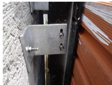
**Figure 10.** Roller support with oblong holes
