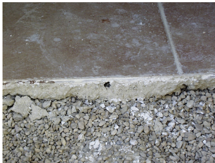
Figure 1. Installation of flooring on gravel and a mortar layer.
