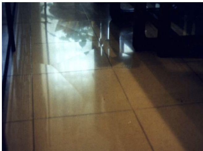
Figure 3. Marble agglomerate flooring with synthetic resins.
