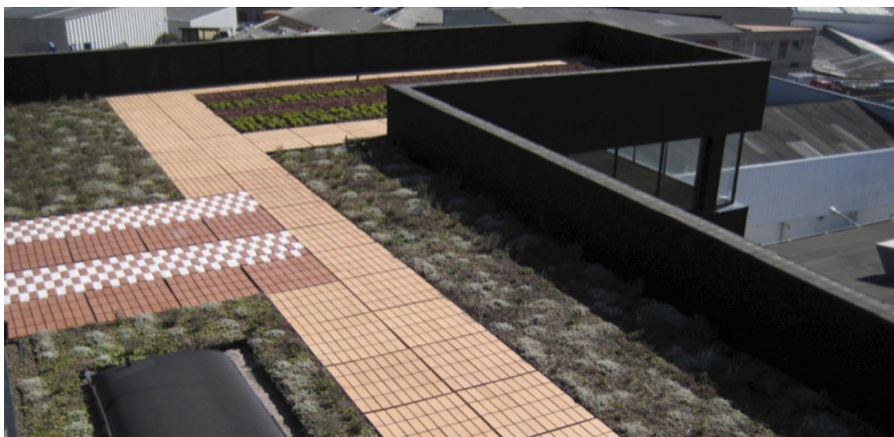
Fig. 4 – Roof Garden on the Giscosa Office Building in Terrassa (archs. Sarrablo and Colom).
