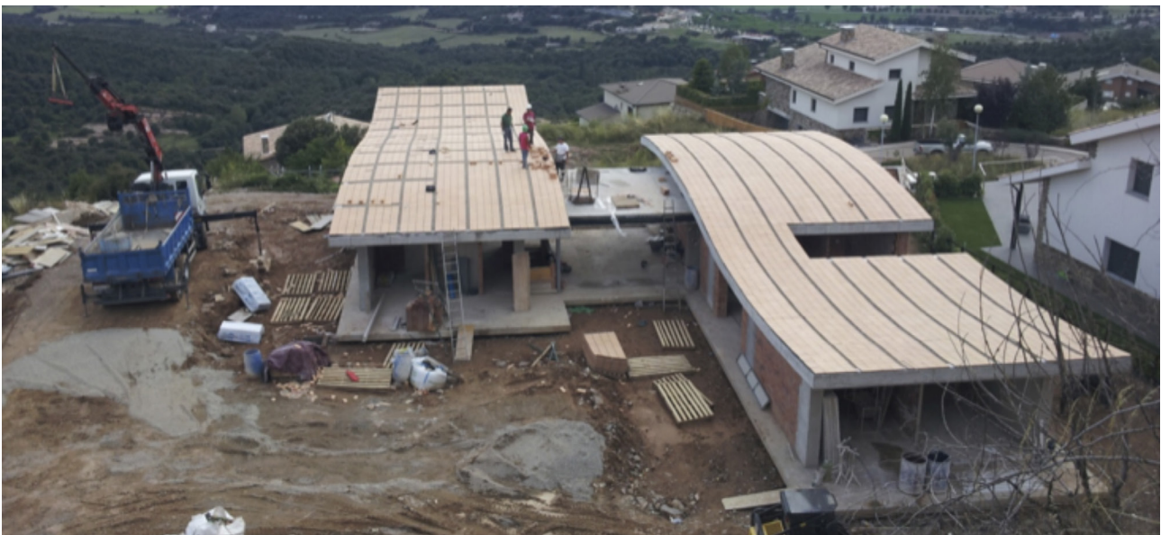
Fig. 8. Building a Curved Roof in Berga (architects Eidee).
