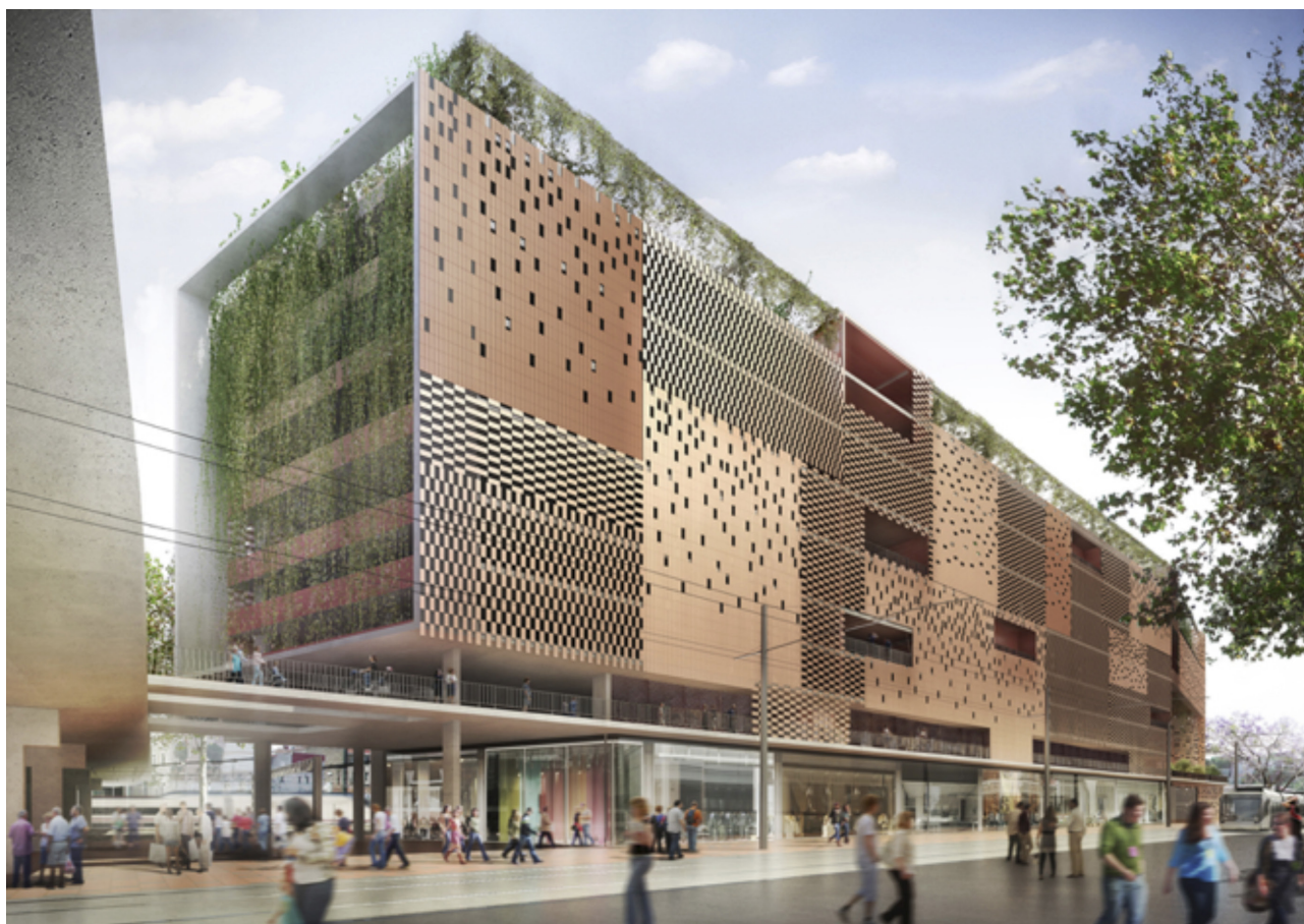
Fig. 13. Saint Roch Car Park in Montpellier (archs. Archikubik).
