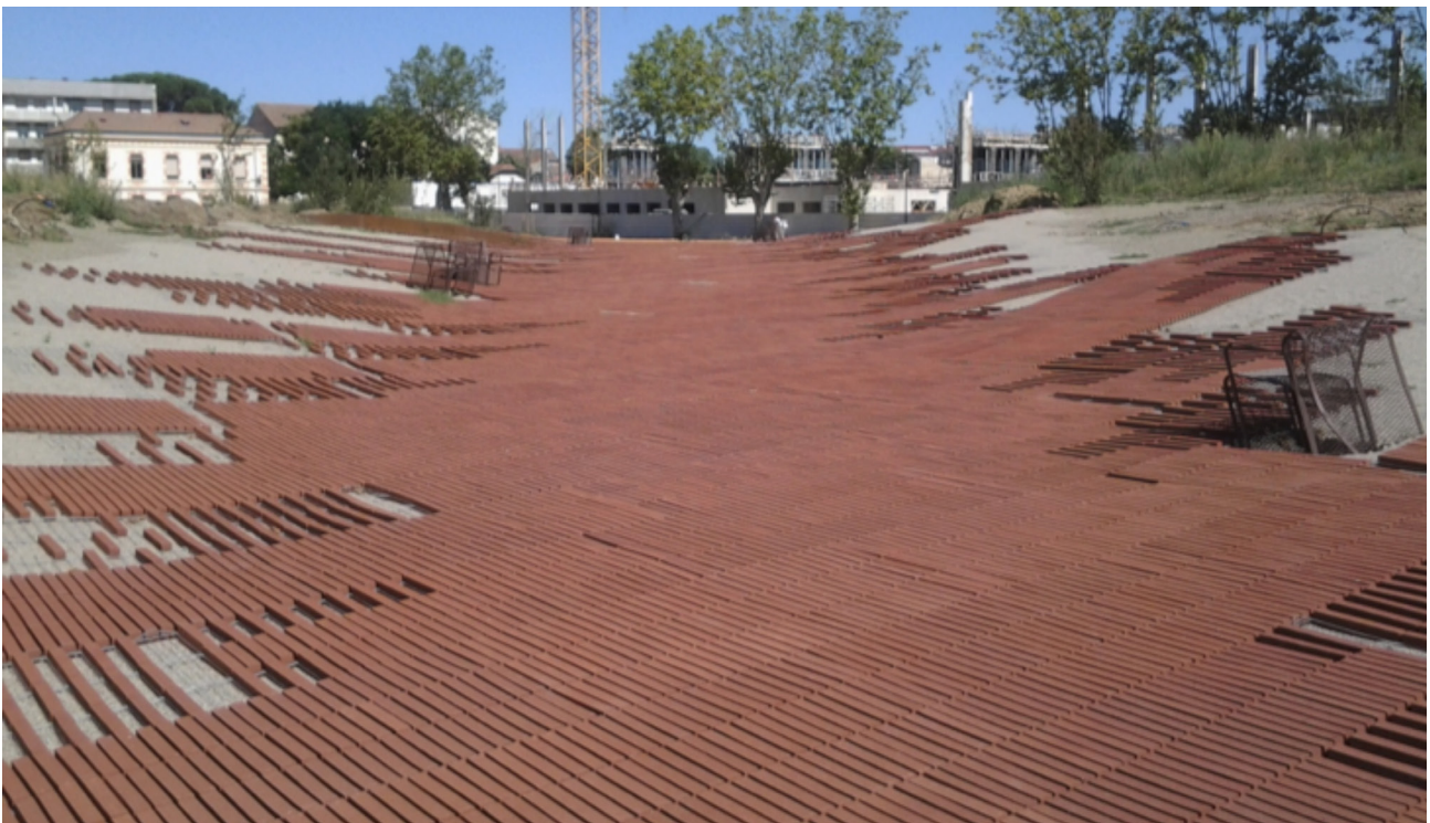
Fig. 3. Execution of the Drainable Paving Project for the Jardín Niel (archs. Michèle & Miquel).
