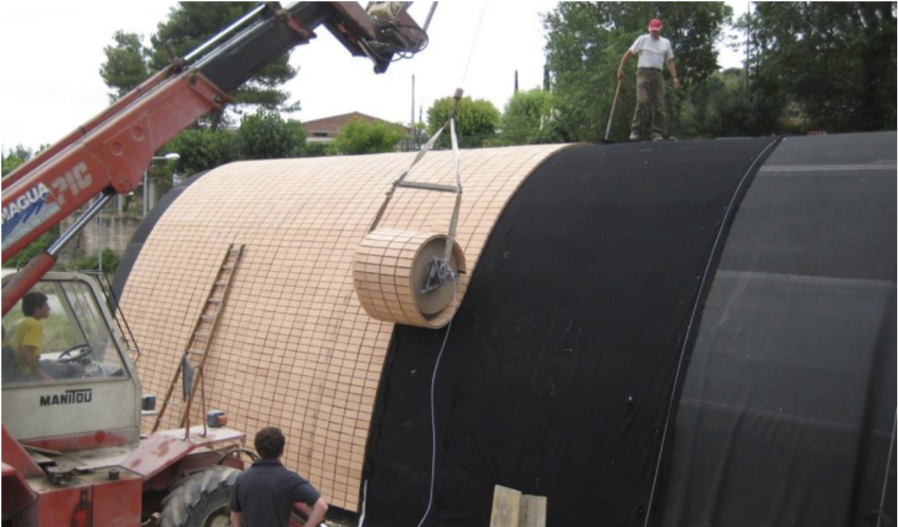
Fig. 7. Covering the Vault for Casa Mingo (architects Sarrablo and Colom).
