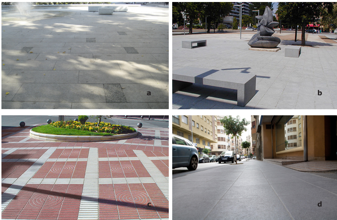
Figure 1. Most common types of urban flooring: a) natural stone slab, b) concrete flag, c) terrazzo tile, d) porcelain stoneware tile.
