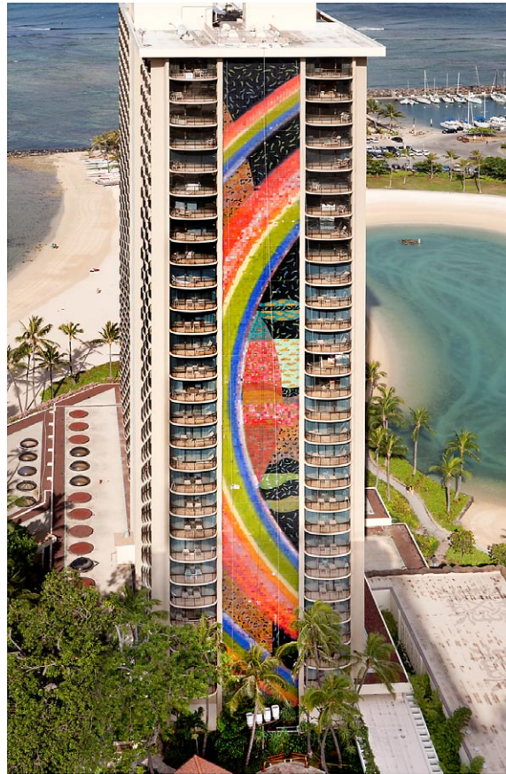
Figure 8 – 30 Story tile façade prior to replacement
