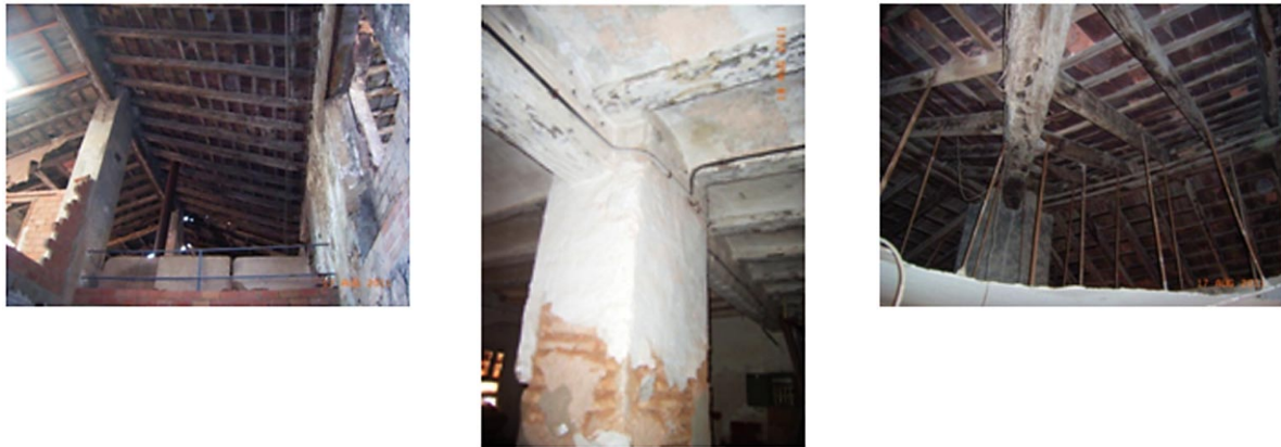
Photos of internal structural components.
