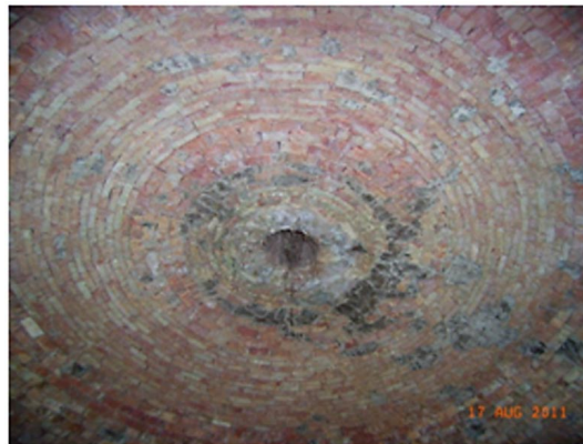
Photo of the roof of the existing kiln.
