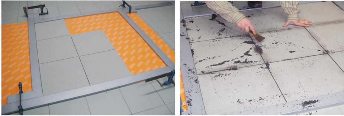
Figure 8. Installation of the powder adhesive system prototype
