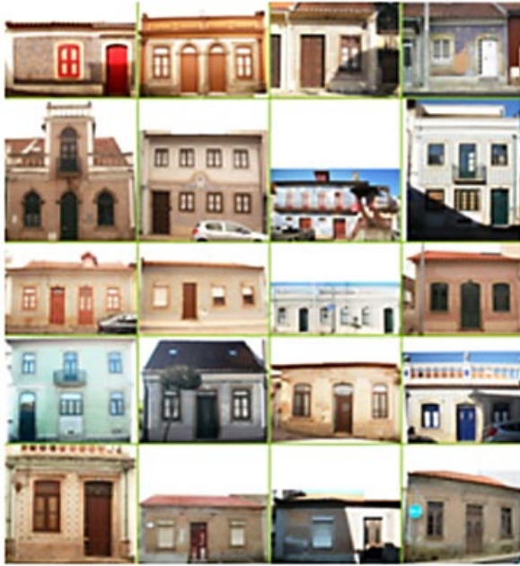
Fig. 1 – Examples of buildings with earthenware tile façades, Ovar.
