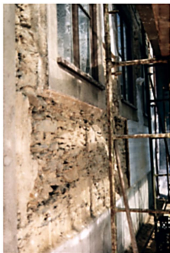
Fig. 3 – Removal of detached tiles during the intervention.
