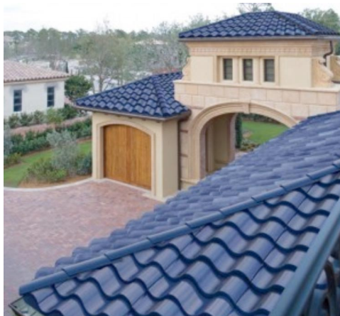
Figure 11. Photovoltaic tiles installed alongside traditional clay tiles. Source: SRS Energy 3 Fuente: SRS Energía 4 .
