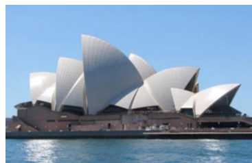
Figure 21. General view of the Sydney Opera House, Australia, Jørn Utzon.
