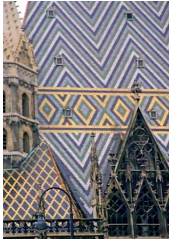
Figure 2. Detailed view of the roof of Saint Steven's Cathedral, Vienna.
