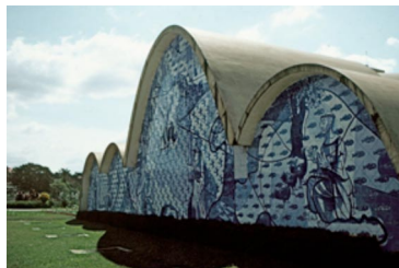
Figure 14. General view of the Saint Francis of Assisi Church, Pampulha, Brazil, Oscar Niemeyer.
