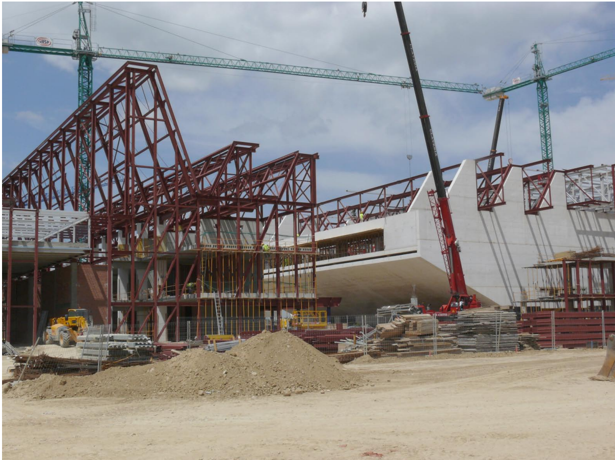
Figure 3. Iron structure of the roof without GRC panels.
