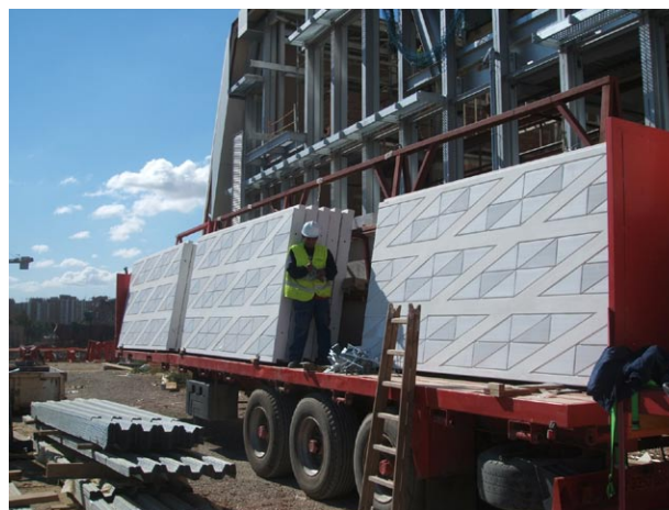
Figure 12. Transport of the panels for their installation.
