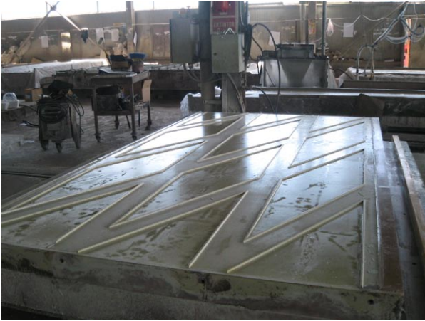
Figure 7. Mould for the fabrication of the GRC panels.
