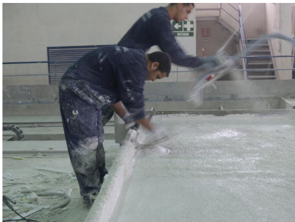
Figure 9. Spraying of cement in the panels.
