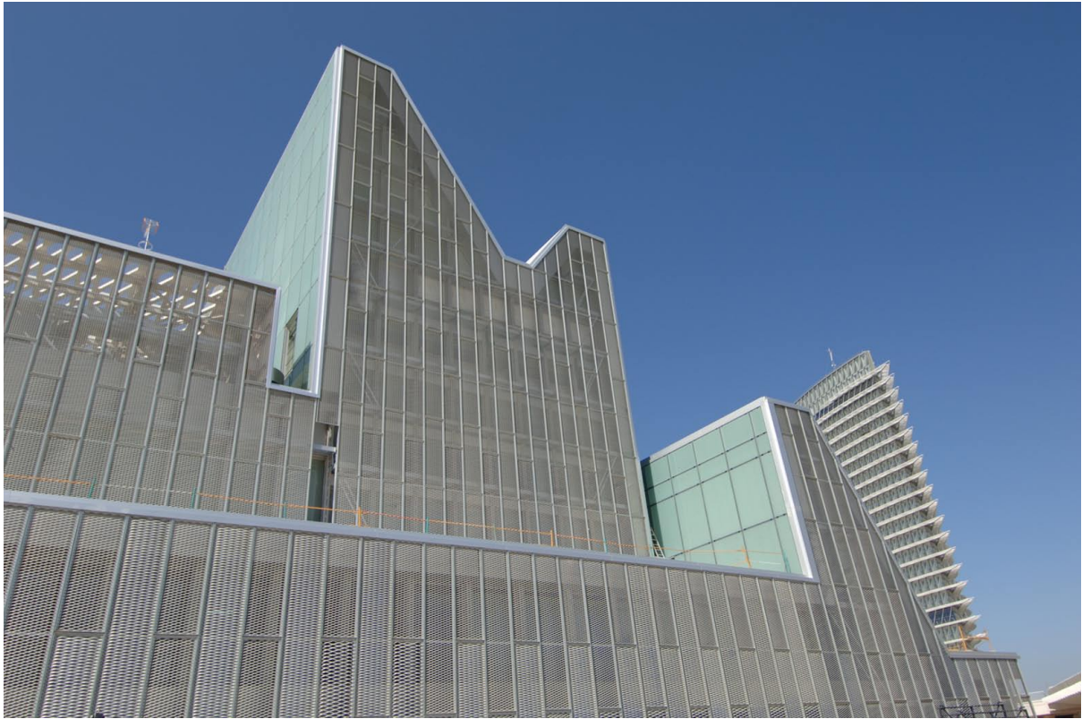
Figure 4. Side view of the skylights.
