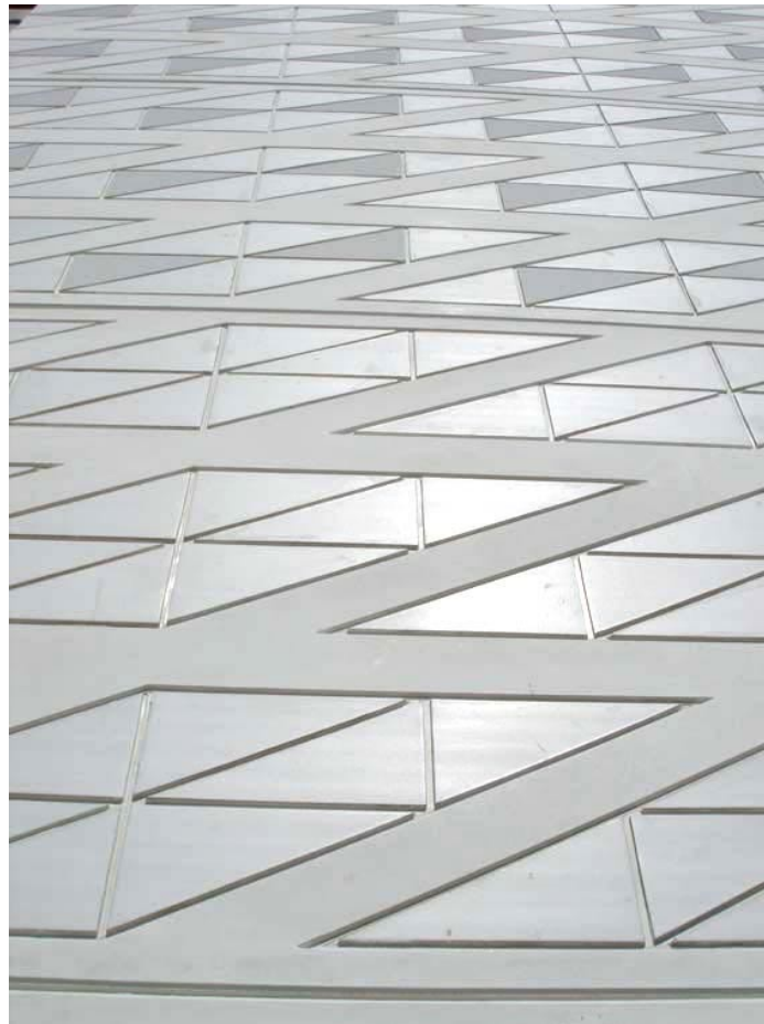
Figure 11. Photograph of the installed roof.
