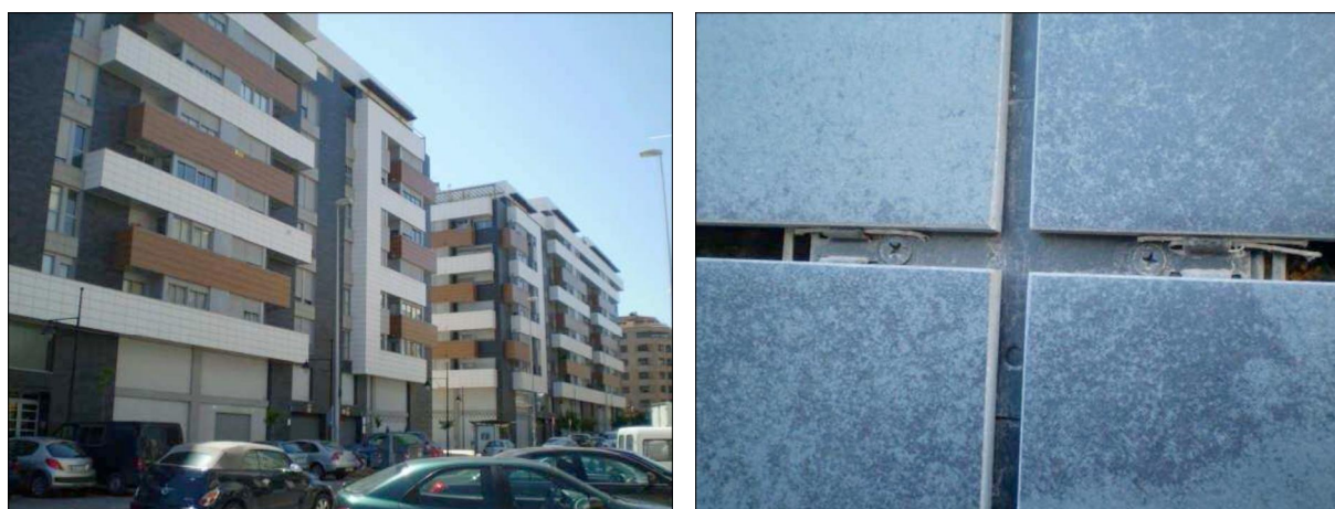
Figure 3. Domech Building. C/ Hermanos Bou no. 44.
