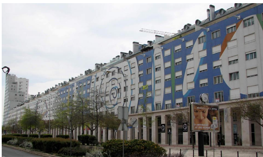
Figure 7. The “Ecran Building”, in Lisbon (2000), may be considered an exception in Portuguese contemporary architecture, in view of the extension of the decorative tile composition and the fact of being mostly a private housing building.
