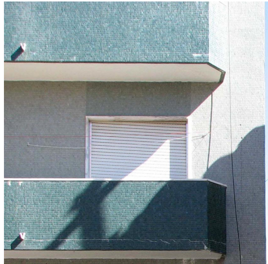
Figure 1. Surface covered with "pastilha" (Sabugal, c. 1970s).
