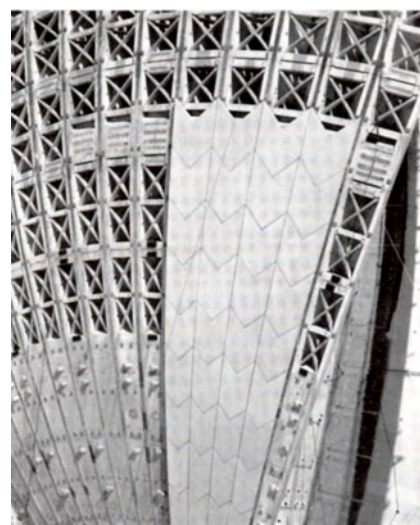
Cladding under construction.
