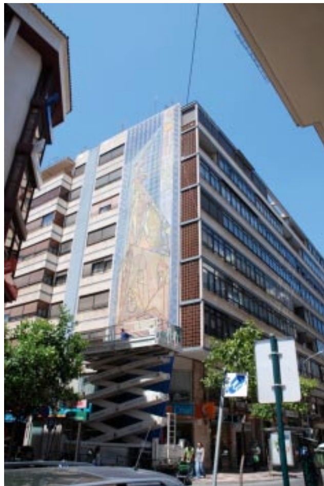
Figure 2. Present view of the building.
