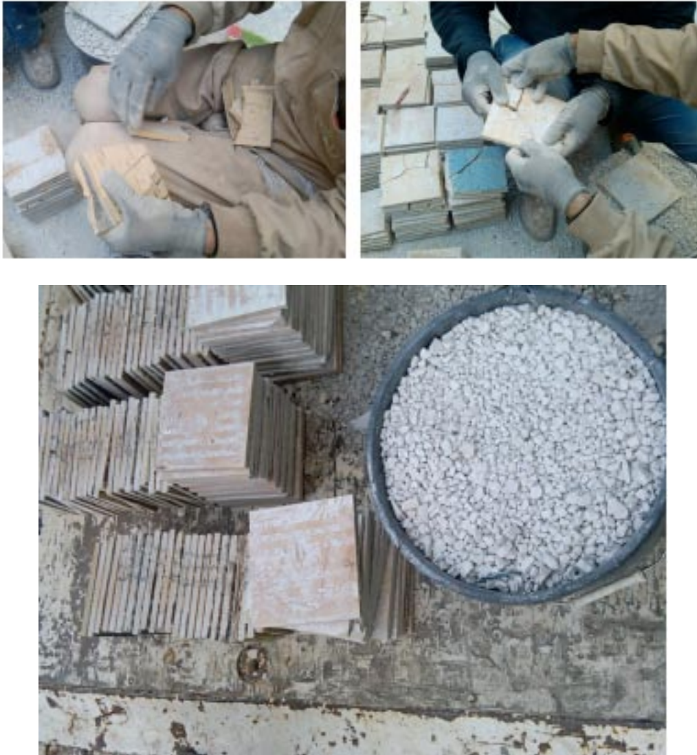
Figure 18. Cleaning and numbering of the original pieces.
