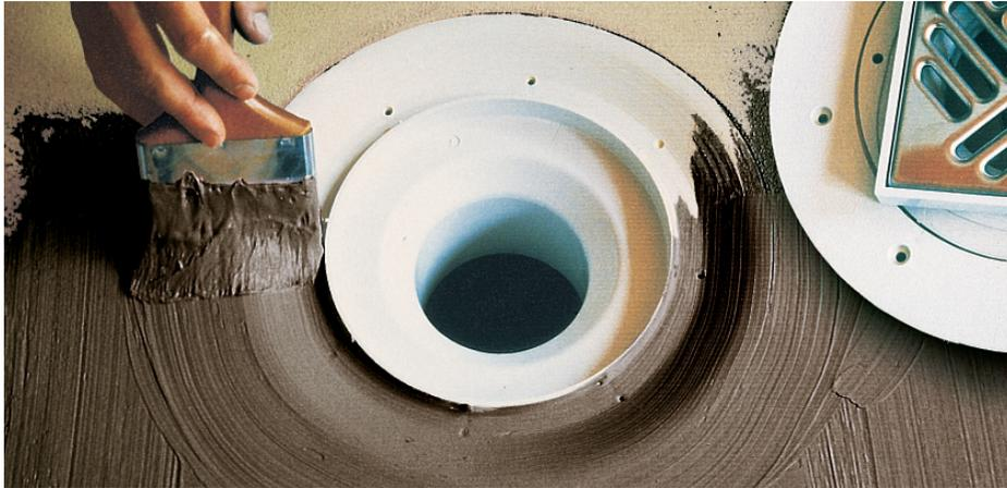
*Figure 1. Coating of the fixed flange with subsequent fitting of the waterproofing gasket into the fresh liquid applied waterproofing*
