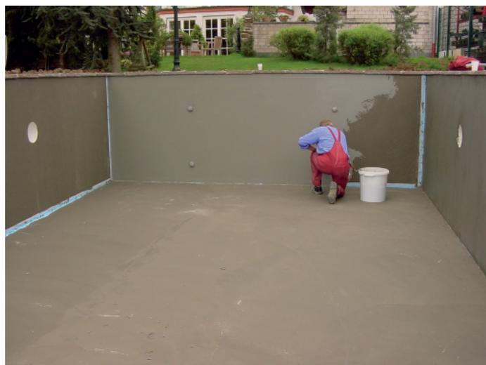
Figure 5. Subsequent coating of the waterproofing tape with a second coat of liquid applied waterproofing
