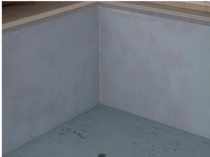
Figure 11. In the case of translucent mosaic in particular, laying and grouting must be carried out using epoxy resin in order to prevent cavities.
