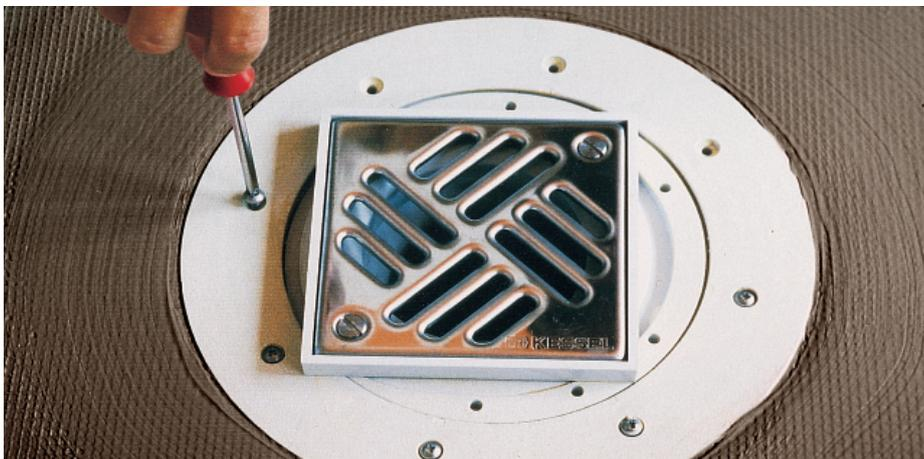
*Figure 3. Bolting of the fixed flange after coating of the waterproofing gasket with liquid applied waterproofing material*
