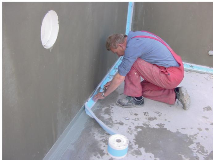
Figure 4. Application of waterproofing tape to the fresh liquid applied waterproofing
