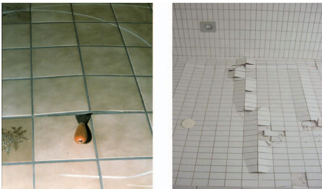
Figure 1. Detachment of ceramic tilings owing to the formation of excessively high stresses
