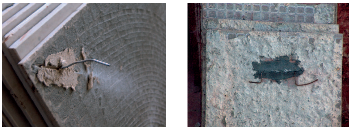
Figure 11. Examples of simple wire anchorage to improve bond stability. Back surfaces of tiles were previously prepared with adhesive mortar or spatter dash.
