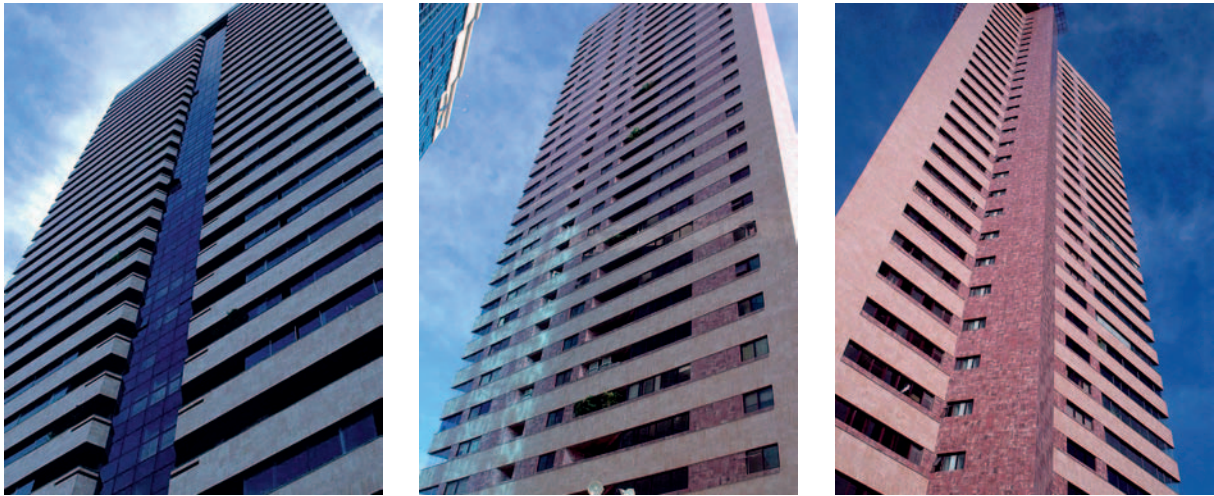
Figure 9. Facade overview of the first great project in Recife where 30 x 30 cm porcelain tiles were used.
