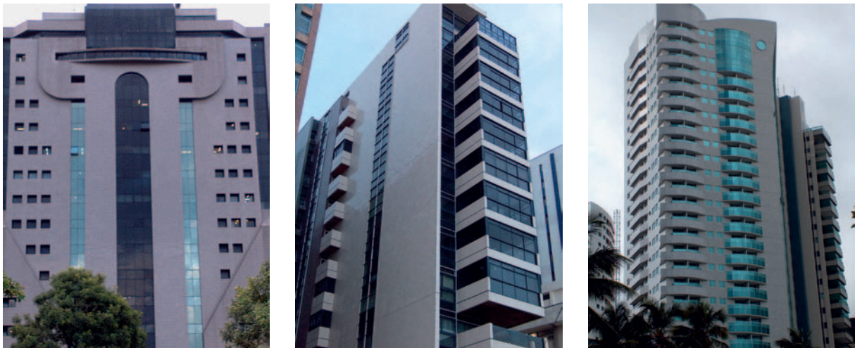
Figure 10. Porcelain tiles building facades in Recife. Most buildings have more than 20 floors. Facades architecture put together ceramic tiles, dimension stone and structural glazing.
