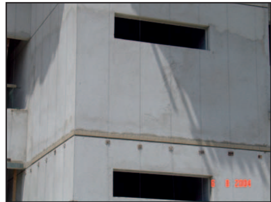
Figure 5. Detail of the horizontal bottom course that enables fastening the vertical reference wires to assure alignment of the pieces throughout the height of the building.
