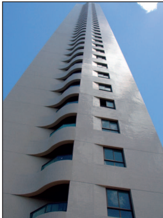
Figure 6. Facade of the Terra Brasilis building with its 46 floors, which stands as a landmark in the urban scenario of the city of Recife in Brazil, concluded in August of 2005.
