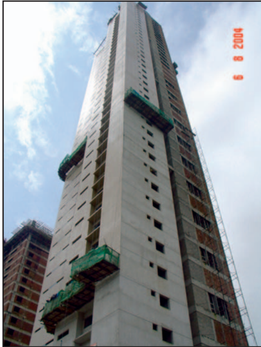
Figure 4. Appearance of the facade during the execution of the render, with access by means of suspended scaffolding. Note the movement joints already installed on all the floors.
