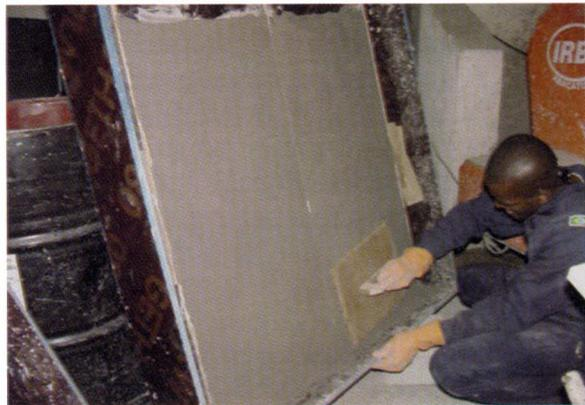
Figure 2. Mortar floating
