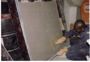
Figure 2. Mortar floating
