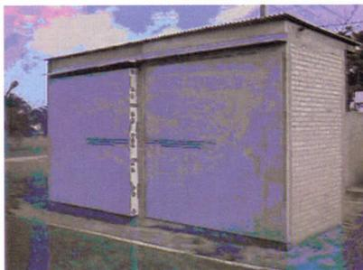
Figure 2. General view of the building with the panels of the ventilated facade prototype and conventional facade.
