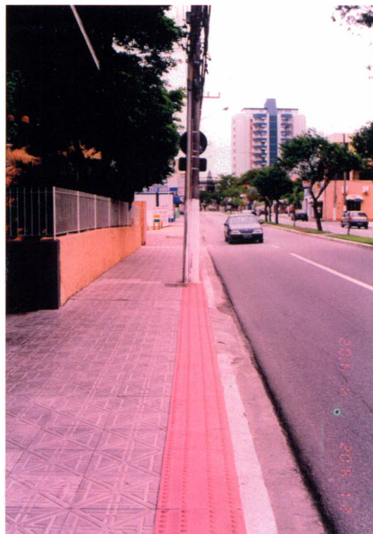
Figure 1. View of a street with alerting flooring in concrete next to the kerb.
