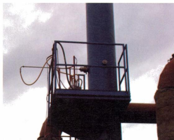
Figure 9. Gas sampling point after the filter.
