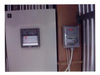
*Figure 7. Detail of the on-line charge loss recording system* ( $\Delta P$ ).
