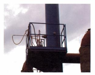
Figure 9. Gas sampling point after the filter.
