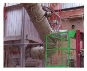
Figure 8. Gas sampling point before the filter.
