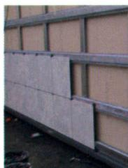
Figure 1: Porcelain tile curtain wall employed as an integrated system with gypsum plasterboards (MÄNTYLÄ, 2002)
