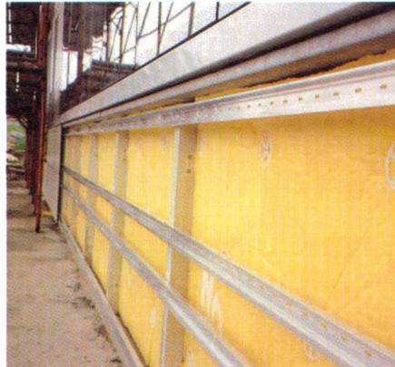
Figure 2: Thermal Insulation (self-standing fiberglass insulating panel) in ventilated facade (MARAZZI, 1997)
