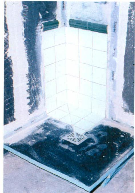
*Prefabrication at the service of the bathroom and kitchen. Extruded closed cell, high density, "Styrofoam"® polystyrene boards covered with fibreglass mesh and cementitious adhesive.
