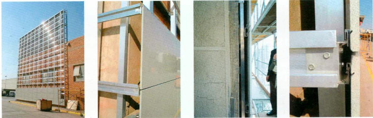
Execution process of a ventilated facade with polished and natural porcelain tile (Dolphin and Coconut series), under the MECANOFAS KARRAT S-7 ® system of auxiliary structure and hidden fastening.
