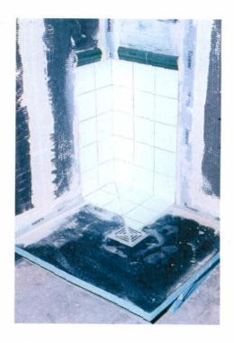
Prefabrication at the service of the bathroom and kitchen. Extruded closed cell, high density, "Styrofoam"®, polystyrene boards covered with fibreglass mesh and cementitious adhesive.
