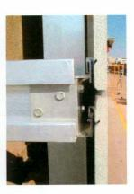
Execution process of a ventilated facade with polished and natural porcelain tile (Dolphin and Coconut series), under the MECANOFAS KARRAT S-7 ® system of auxiliary structure and hidden fastening.
