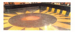
Large slabs of terrazzo and continuous flooring at Bilbao airport Continuous agglomerate flooring. INYETPAVI® system . Photo: Baltanás, Sánchez SOURCE: ON DISEÑO, nº. 221, pág. 374.
