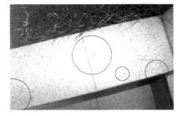
Figures 10, 11: Frost damage to dry-pressed glazed ceramic tiles in situ.
