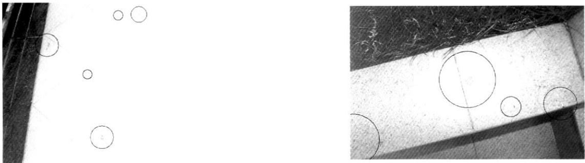
Figures 10, 11: Frost damage to dry-pressed glazed ceramic tiles in situ.
