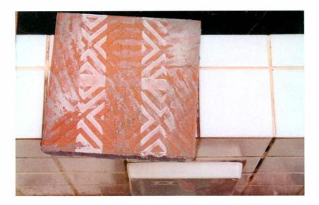
Figure 6: Evidence of the lack of coverage on the back of the ceramic tiles.
