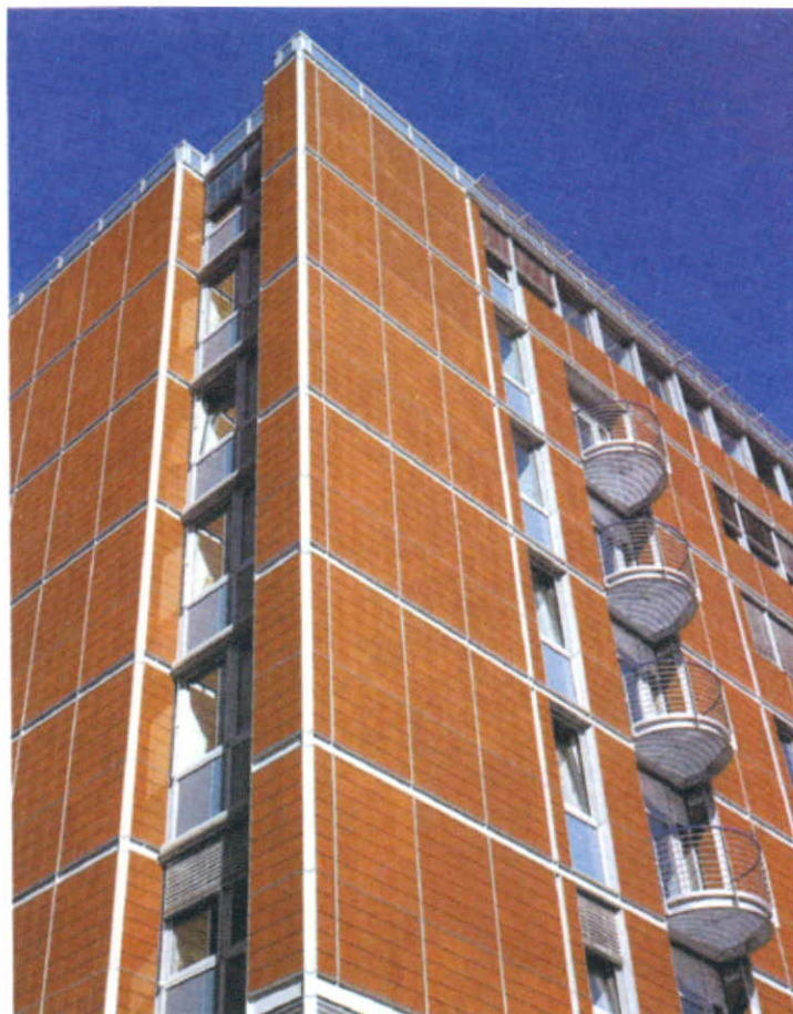
Figure 20 - Service Center Ostkreuz, Berlin – example of ventilated tile system using prefabricated panels 3 m x 7.5m wide which emphasize technical details of panel frame and tile attachment.
