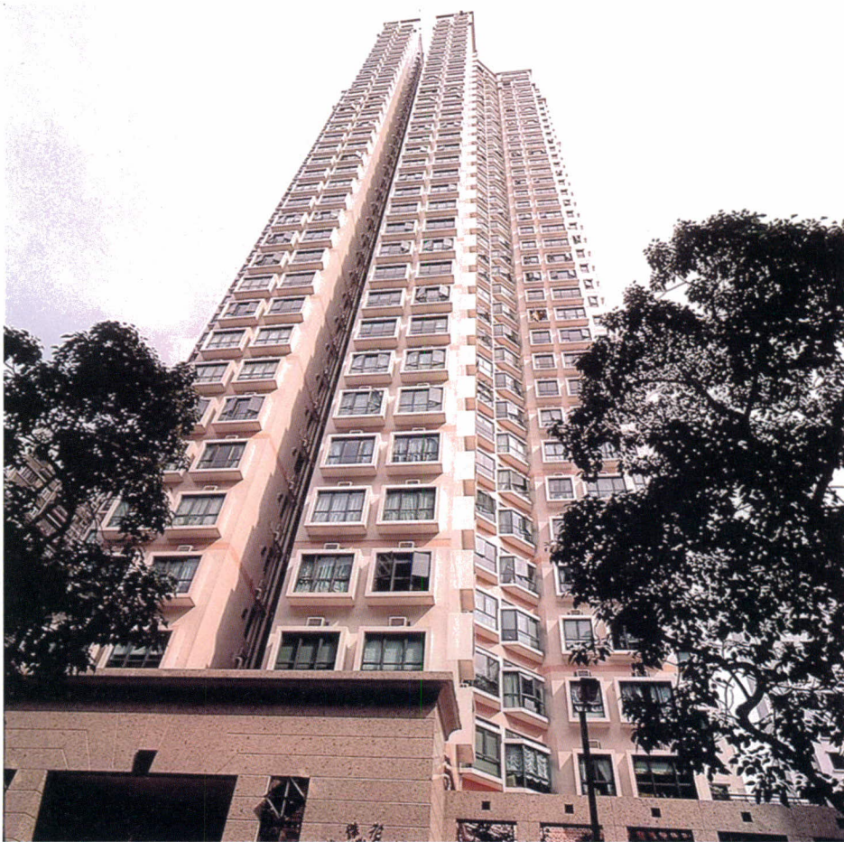
Figure 2 - 3 Babington Path residential high rise project in Hong Kong clad in-situ with ceramic mosaic tile adhered with latex cement adhesive.
