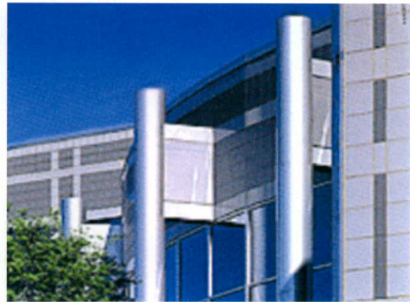
Figure 10 - Naval Intelligence Center, Suitland, Maryland, USA incorporating prefabricated ceramic tile clad panels with tile adhered by structural silicone adhesive.
