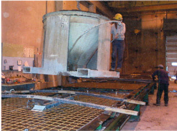
Figure 15 - Placement of concrete over tile and steel reinforcing.
