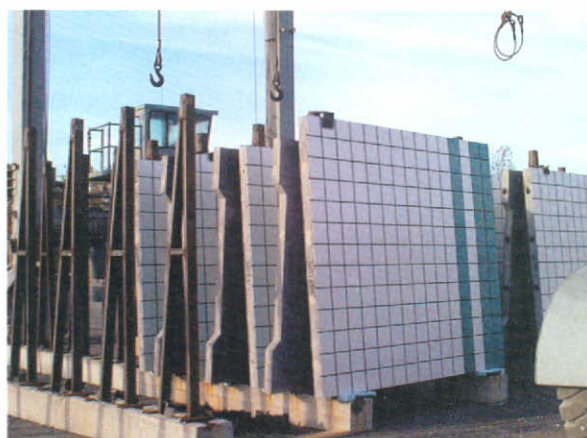
Figure 13 - Panels hoisted into place at site.
