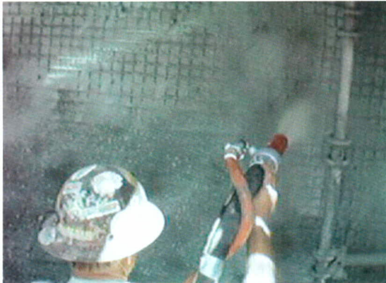
Figure 8 - Pneumatic application of latex cement render over steel wire mesh secured to reinforced concrete with stainless steel anchors.
