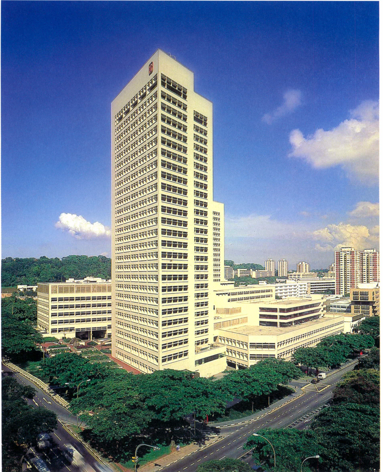
Figure 3 - The Housing Development Board Building, Singapore, clad with 150 x 150 mm ceramic tile and installed in-situ with latex cement adhesive.
