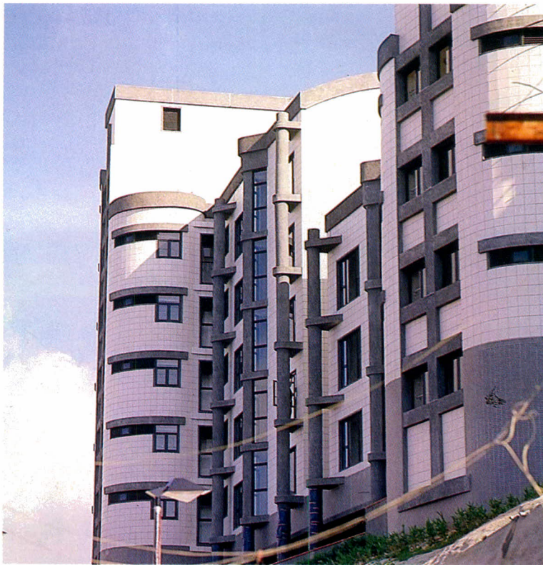
Figure 4 - Residential project at the Cloudlands and Cliff at the Peak in Hong Kong, PRC, an example of an in-situ tile clad façade, adhered with latex cement adhesives.
