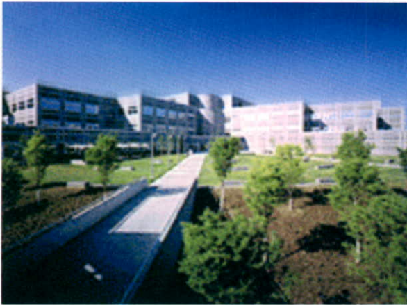
Figure 10 - Naval Intelligence Center, Suitland, Maryland, USA incorporating prefabricated ceramic tile clad panels with tile adhered by structural silicone adhesive.
