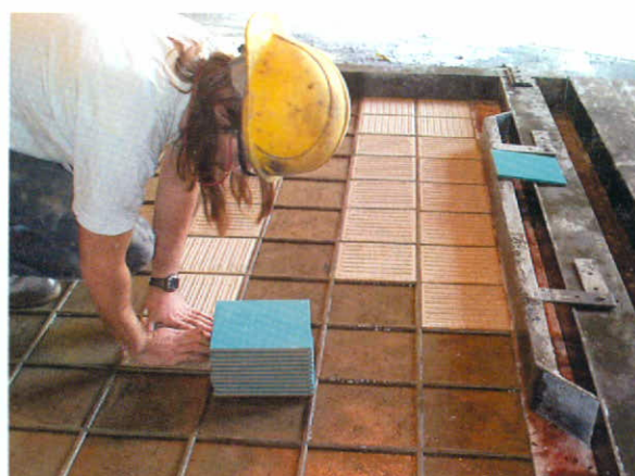
Figure 12 - Placing key back tile face-down into the precast concrete panel mold.
