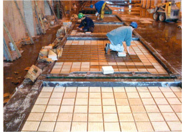
Figure 16 - Large-scale production capabilities for tile installation.
