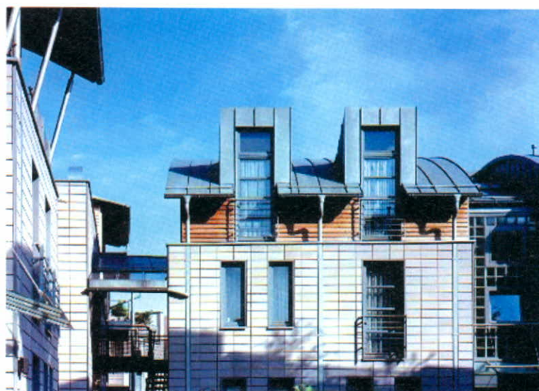
Figure 21 - Example of current trend towards architectural expression of technology using zinc metal and ventilated tile façade mechanically attached in-situ.
