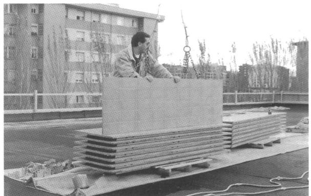
*Figure 17. Installing a backing panel.*
