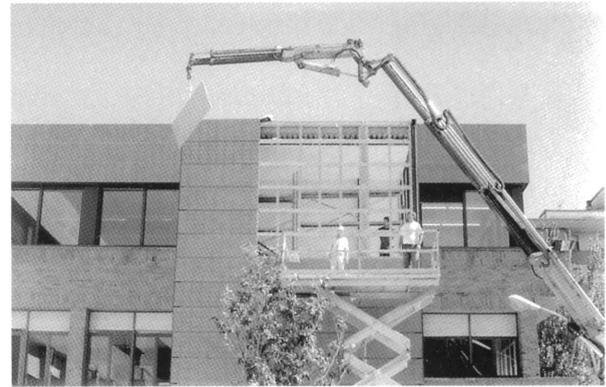
*Figure 21. Installation of Model 2 panels on the stair.*
