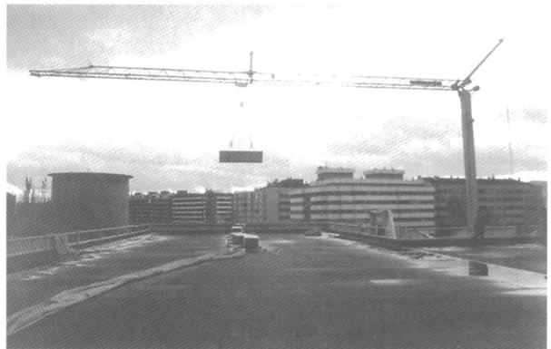
*Figure 13. Hoisting the elements onto the roof.*
