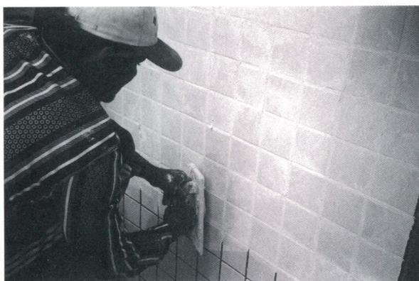
*Figure 15. A rubber trowel designed for jointing is used here for adequate filling.*
