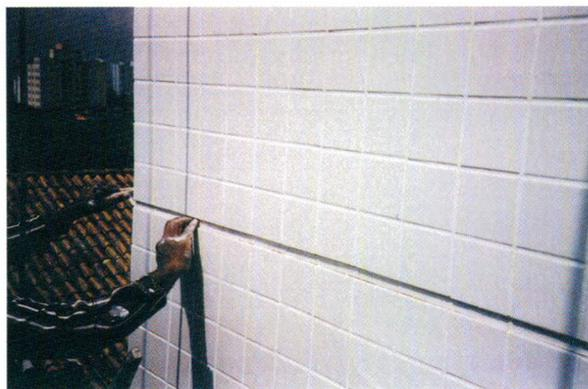
*Figure 18. Back-up tape is used to avoid sealant bonding to the back of the control joint. The technique is essential to sealant behaviour and durability.*
