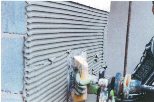
*Figure 10. The notched edge of the trowel is used to prepare the surface for adequate fixing. Horizontal stripes are preferable to avoid eventual water leakage.*
