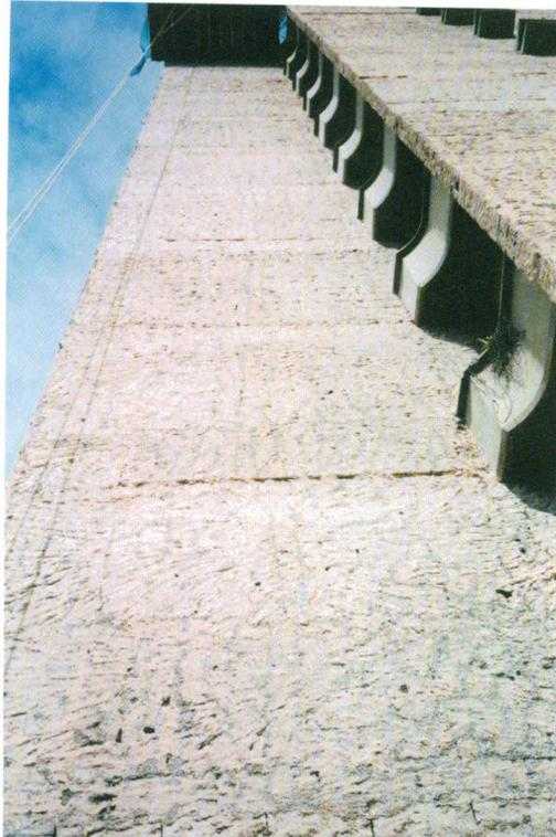
*Figure 6. View of facade where old ceramic tiling has been removed. Surface cleaning was necessary to allowing bonding new layers.*
