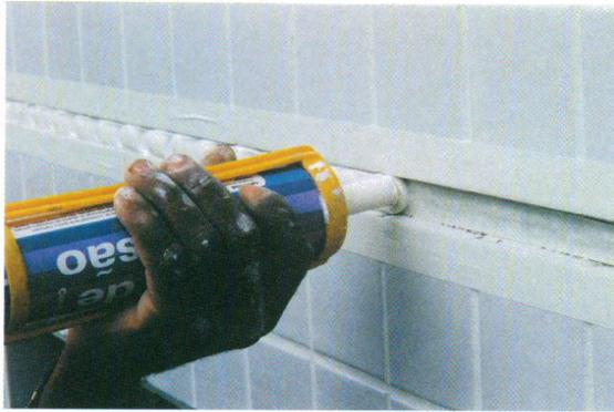
Figure 19. Sealant is applied in the control joint. Jointing is necessary after the preset time of the material. Note that tape used to protect tile edges.
