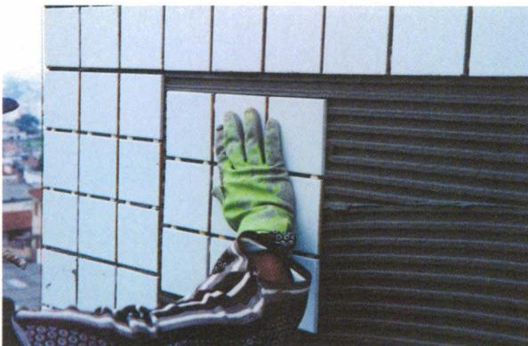
*Figure 11. Tiles are positioned by offsetting them from their final place so the adhesive can be fully spread. The technique is very simple but gives good results to improve coverage.*
