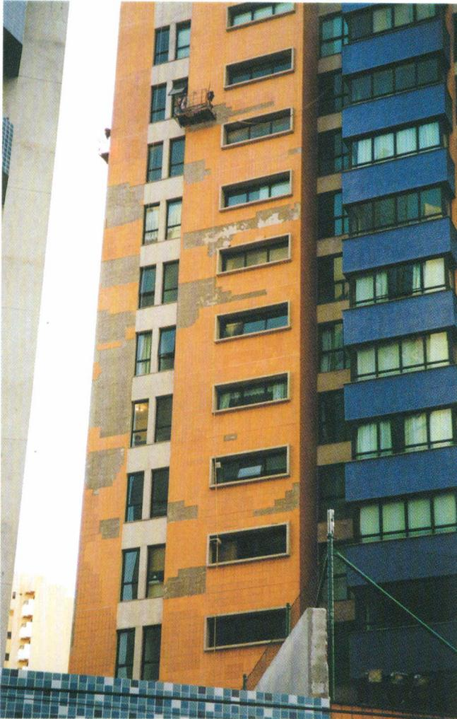
*Figure 1. View of building facade where the bond between adhesive and tile broke. Correction requires removing of tiles and preparation of surface when cement-sand rendering remains adequate.*
