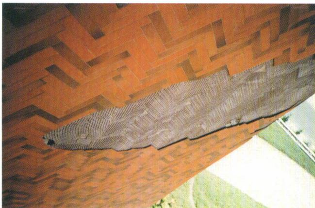
*Figure 2. Detail shows bond installation problem but tiling also presents inadequate joint thickness, no control joint and very rigid adhesive mortar and grout.*
