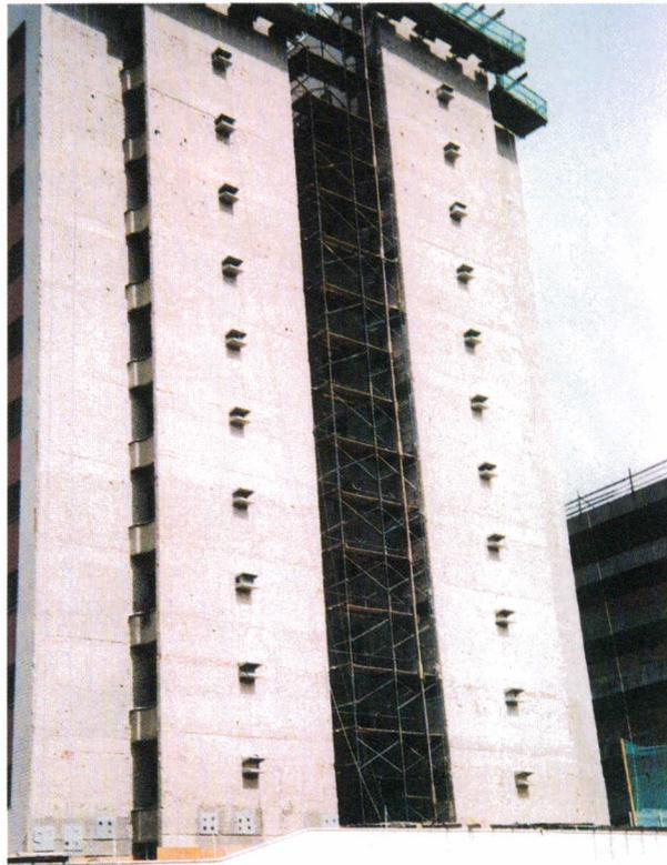
*Figure 4. Cement-sand render substrate shows rupture. Inadequate specification of mortar was considered main cause here. Creep of concrete framework and differential movements of masonry infilling contribute to the situation. There were horizontal joints but they were incorrectly positioned.*
