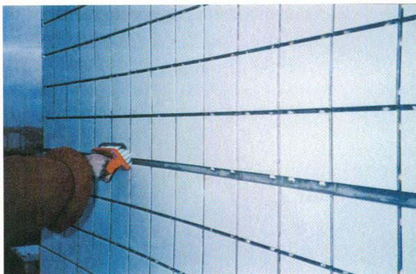
*Figure 13. Joint cleaning is very important to let the grout fill the joints completely. Here a brush is used.*
