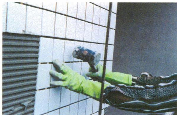
*Figure 12. The tiles are pressed against the background, not only to improve coverage but also to prevent slipping. The material is isotropic and squeezes when pressed by percussion.*
