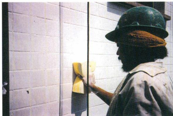
*Figure 16. Primary cleaning of grout that spills out of the joint and remains on the surface of tiles. A sponge is used.*
