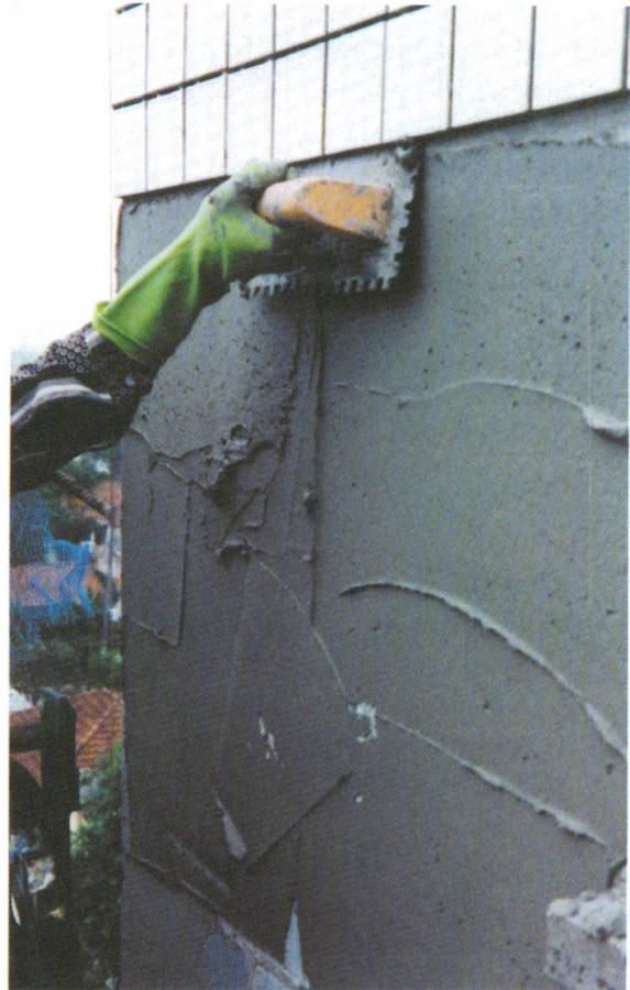
*Figure 9. Adhesive mortar is spread first with the flat edge of the trowel to guarantee coverage of the background. In this case, a square shaped, 8mm height notched trowel was used.*
