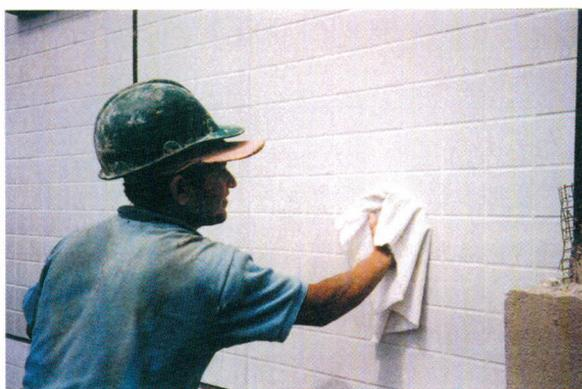
*Figure 17. Secondary cleaning of the tiling surface. Beyond this step only final cleaning is required.*
