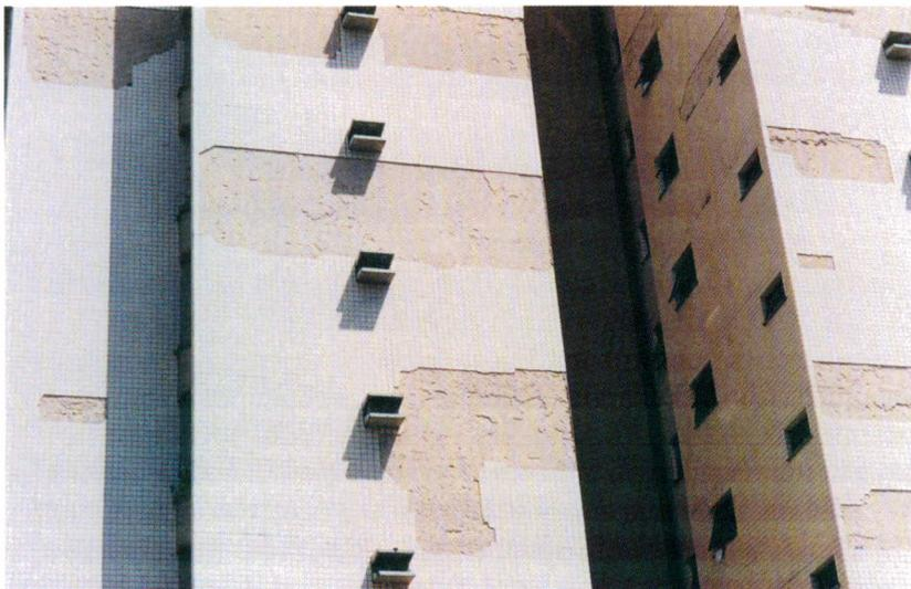
*Figure 5. Here the entire system has been removed. This costs about 100 % more than initial costs but there was no other way to fix the problem.*
