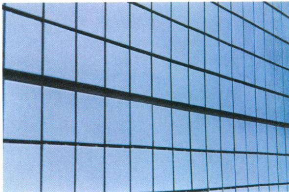
*Figure 14. View of the cleaned ceramic tiling, ready for the application of joint grout.*
