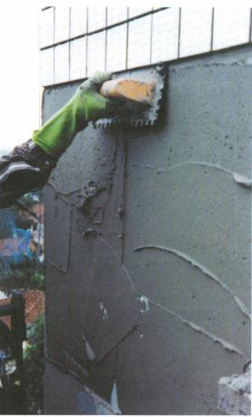
Figure 9. Adhesive mortar is spread first with the flat edge of the trowel to guarantee coverage of the background. In this case, a square shaped, 8mm height notched trowel was used.
