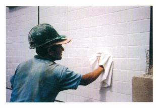
Figure 17. Secondary cleaning of the tiling surface. Beyond this step only final cleaning is required.
