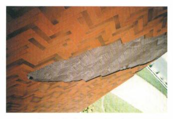
*Figure 2.* Detail shows bond installation problem but tiling also presents inadequate joint thickness, no control joint and very rigid adhesive mortar and grout.
