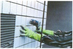
*Figure 12.* The tiles are pressed against the background, not only to improve coverage but also to prevent slipping. The material is isotropic and squeezes when pressed by percussion.
