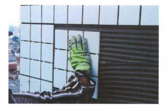
Figure 11. Tiles are positioned by offsetting them from their final place so the adhesive can be fully spread. The technique is very simple but gives good results to improve coverage.
