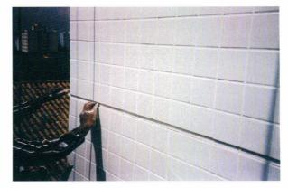
Figure 18. Back-up tape is used to avoid sealant bonding to the back of the control joint. The technique is essential to sealant behaviour and durability.
