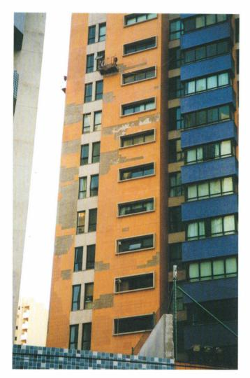
Figure 1. View of building facade where the bond between adhesive and tile broke. Correction requires removing of tiles and preparation of surface when cement-send rendering remains adequate.
