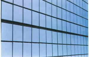
*Figure 14.* View of the cleaned ceramic tiling, ready for the application of joint grout.
