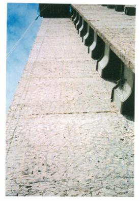
Figure 6. View of facade where old ceramic tiling has been removed. Surface cleaning was necessary to allowing bonding new layers.
