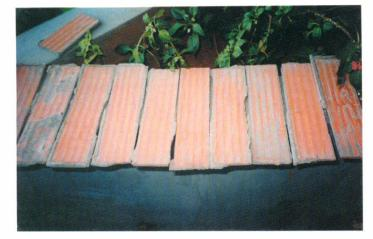
**Figure 3.** Tiles removed from the facade show problem of fixing. Inadequacy of setting together with wrong specification of material caused failure.
