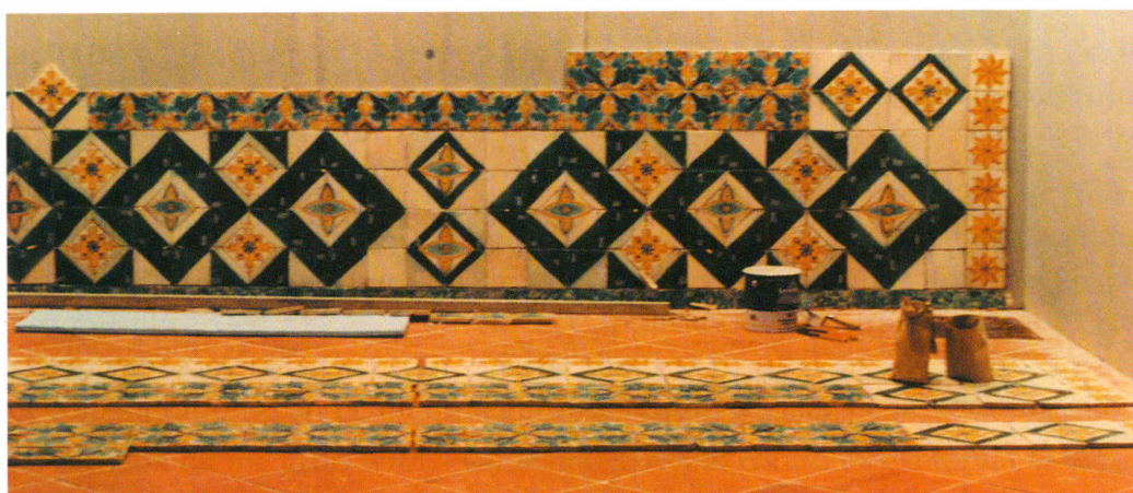
Preparation of the walls, insulation and tile assembly in situ.
