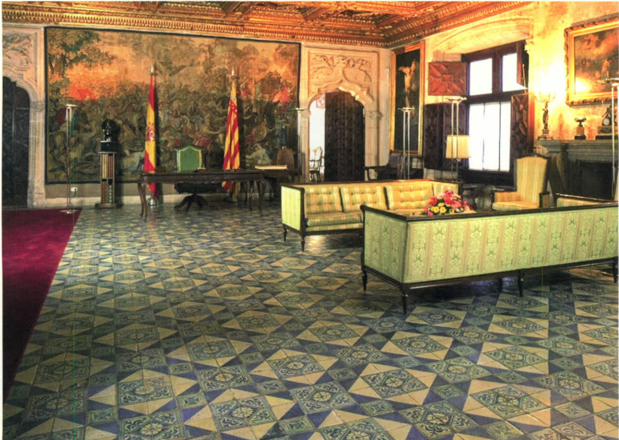
Flooring in the Sala Dorada of the Palace of the Generalitat Valencia, built in the 30s, with serious preservation problems.
