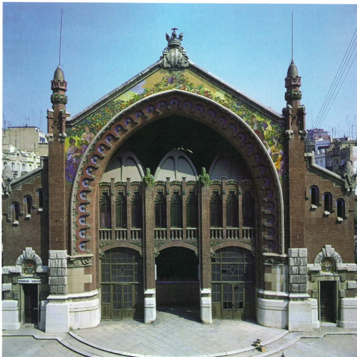
Outside view of the Colon Market, currently awaiting restoration.
