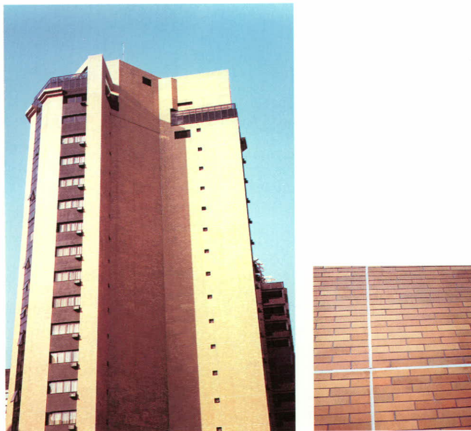
Figure 4. Façade of a building where ceramic tile design has been used with success. Detail shows vertical and horizontal control joints.
