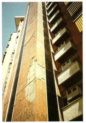
Figure 2. General failure of ceramic tile façade. Extruded stoneware were used with an ordinary mortar. Weather conditions during summer are very severe. Temperature above 40°C is usual. Control joints were built after the bond had failed.
