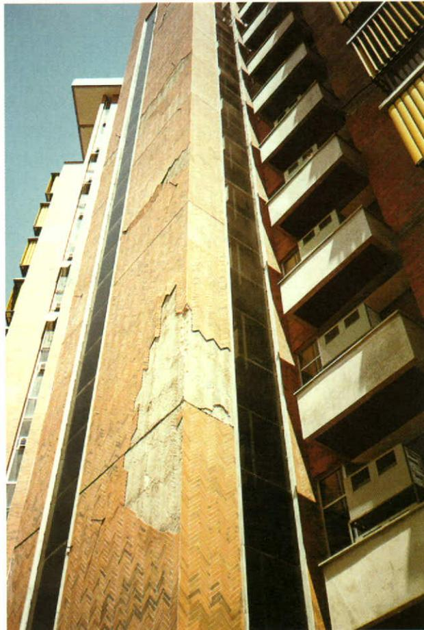
*Figure 2. General failure of ceramic tile façade. Extruded stoneware were used with an ordinary mortar. Weather conditions during summer are very severe. Temperature above 40°C is usual. Control joints were built after the bond had failed.*
