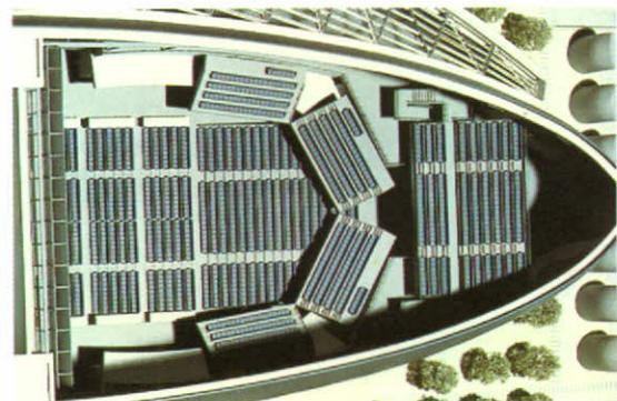
*Seat layout in the "End-Stage Type". The stage boxes on the first floor move on rails in a circle. The stall seats move by a compressed air bearing system. The proscenium has an elastic capacity and allows the stage depth to be adjusted.*
