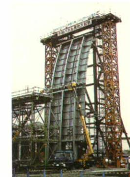
*State of the building with the "Panta dome" system. It lasted 5 days, starting on 1 December 1997.*
