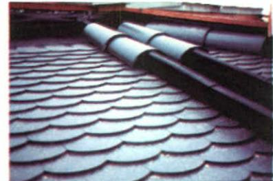
*Chipboard painted like ceramic tiling was used as a sample to test the size, shape and installation system.*
