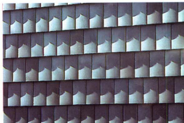
*Shadow test using sunlight. The centre region of the tile has slightly convex design so that natural light will enrich its expression.*
