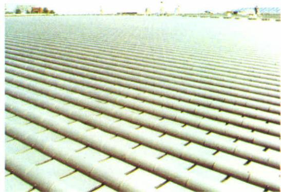
*The almost horizontal roof of the congress and convention halls is covered with tiles installed on stainless steel sheeting that acts as a sealing, providing thermal and acoustic insulation, while keeping in harmony with the surrounding landscape.*
