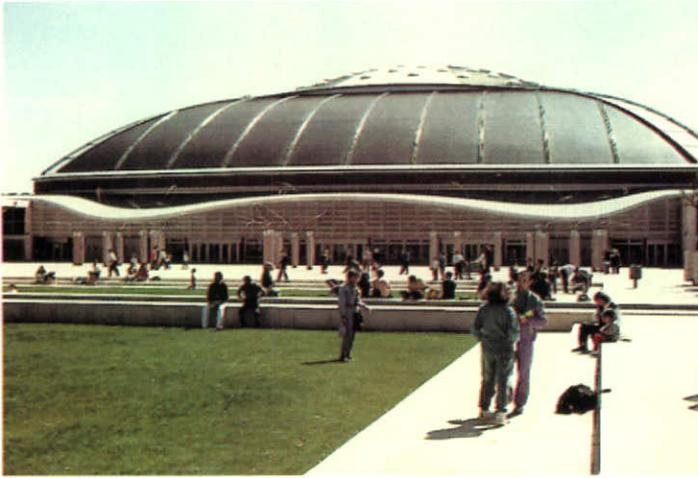
*Ceramic tiles were used on the main roof, and zinc tiles were employed on the low roof.*
