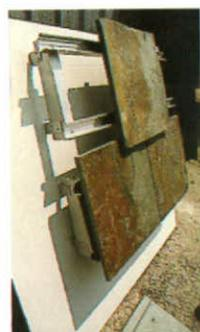
to use slate, an autochthonous material in Galicia, one of the main slate producing regions. Galician slate has an exceptional quality and low cost, which is why the whole facade of the clothoid curve was built with prefabricated concrete panels, onto which grey-greenish coloured slate tiles were hung by iron fastenings. Another screen-shaped wall located at the back is made of granite blocks with light concrete reinforcement.
