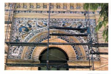
30. Left side of the building, left tower. Appearance after finalising the intervention. Besides the work done on the tiling, the stucco restoration can be observed, imitating brickwork in the arch curve.
