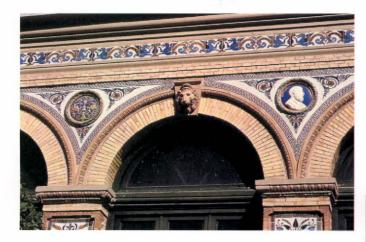
20. The same part, after the intervention: restored tiles, recovery of the original polychromatic colouring of the plaster mouldings: and texture of the keys and ova mouldings of baked clay.
