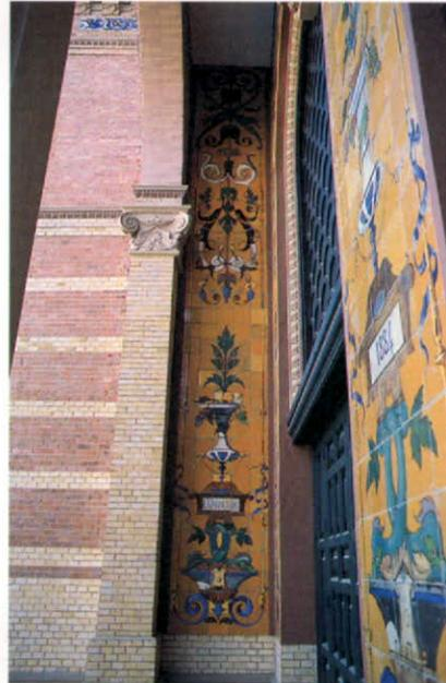
30. Left side of the building, left tower. Appearance after finalising the intervention. Besides the work done on the tiling, the stucco restoration can be observed, imitating brickwork in the arch curve.
