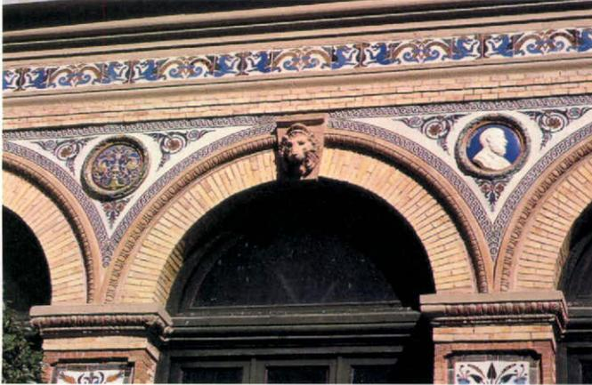
20. The same part, after the intervention: restored tiles, recovery of the original polychromatic colouring of the plaster mouldings: and texture of the keys and ova mouldings of baked clay.
